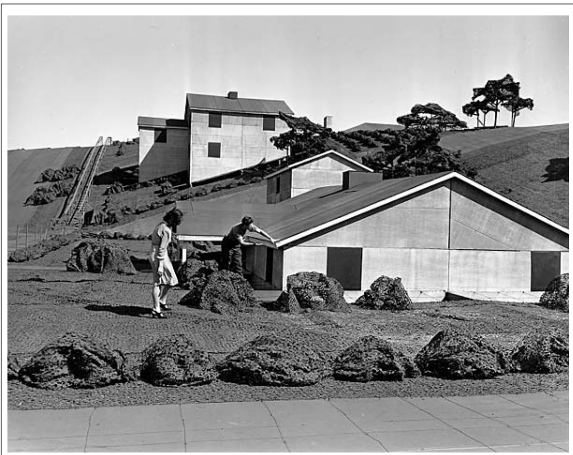
Figure 1-2. Boeing Company Workers Camouflage the Seattle Factory to Look like a Residential Neighborhood from the Air (1942) (© Boeing Corporation)
